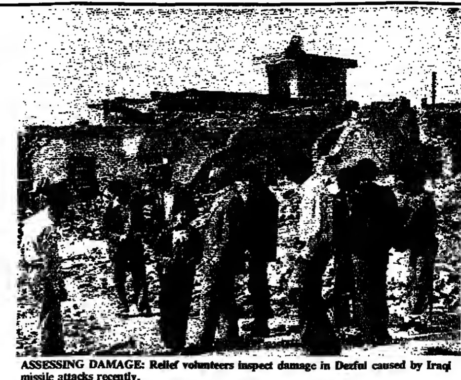
ASSESSING DAMAGE: Relief volunteers inspect damage in Dezful caused by Iraqi missile attacks recently.
